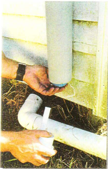
Ball in downpipe rises to block pipe.
