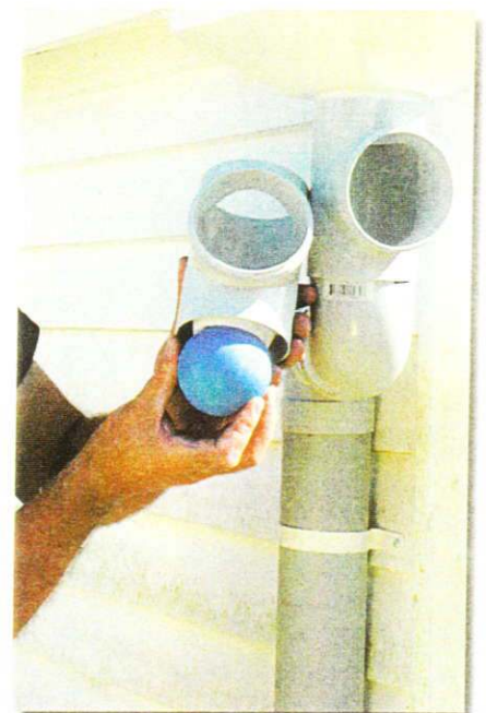
How ball blocks top of first flush diverter.
